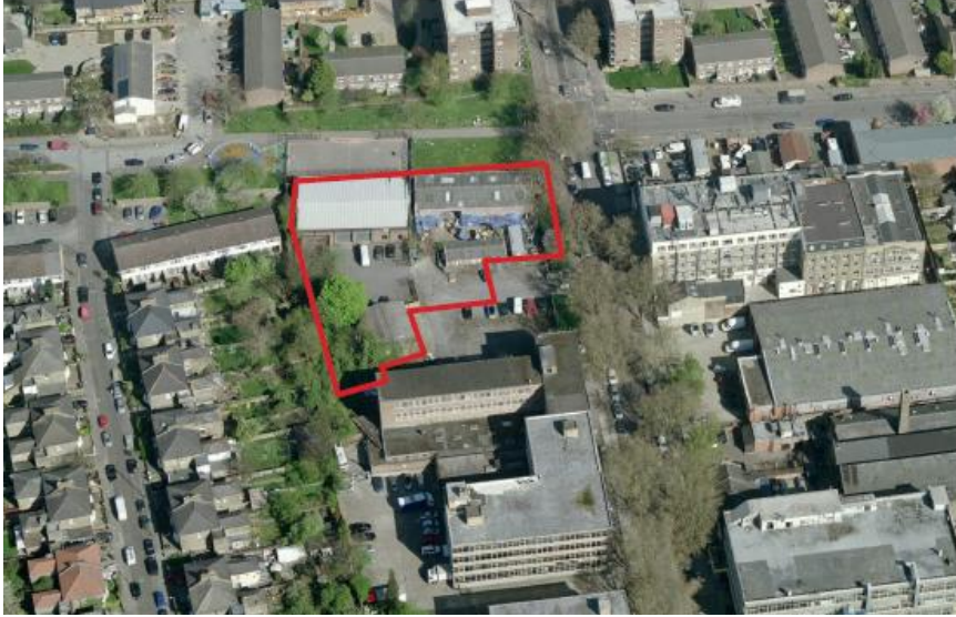
Aerial view – 45-63 Lawrence Road
